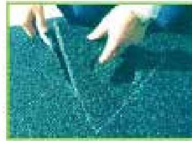
Cut back area neatly with knife to give a clean edge
