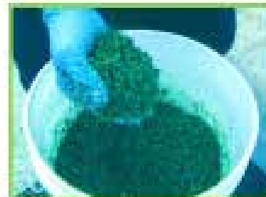
Mix the granules and polyurethane binder together in the bucket
