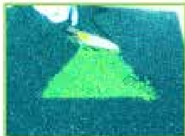
Screed and compress granules into the area
