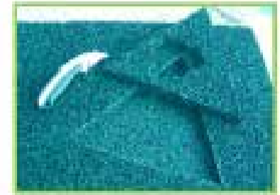
Remove damaged area
