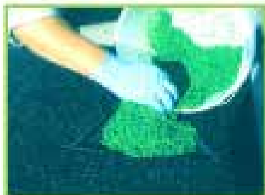
Overfill the hole to allow for compression
